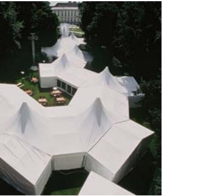
RÖDER solutions are fastened with anchors that do not require a foundation. The unique "heavy floor" technology allows large buildings to be installed without damaging the material. It is possible to assemble a frame tent on any surface.
